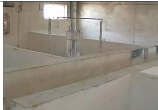
A room fully lime washed
