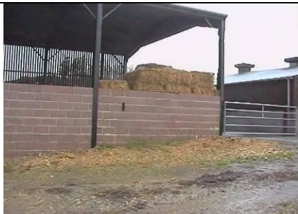
Straw stacks need rodent control programmes
